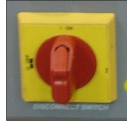
Figure 3. Disconnect Switch.
