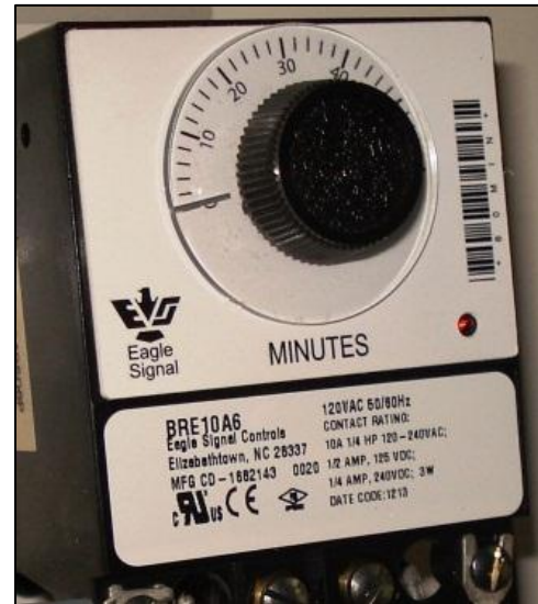
Figure 10. The Purge timer red light is illuminated during the timing period.
